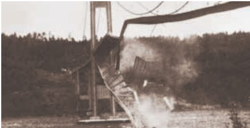
Figure 8.4 Resonance produced such violent vibrations in the original Tacoma Narrows Bridge that it collapsed.
